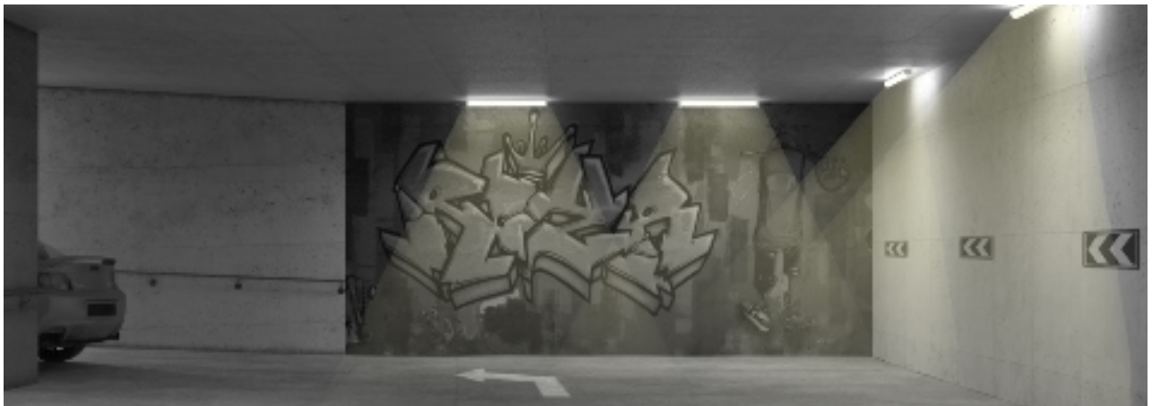
If lamp hasn't detected movement of object, after hold time the lamp will dim to a low level
